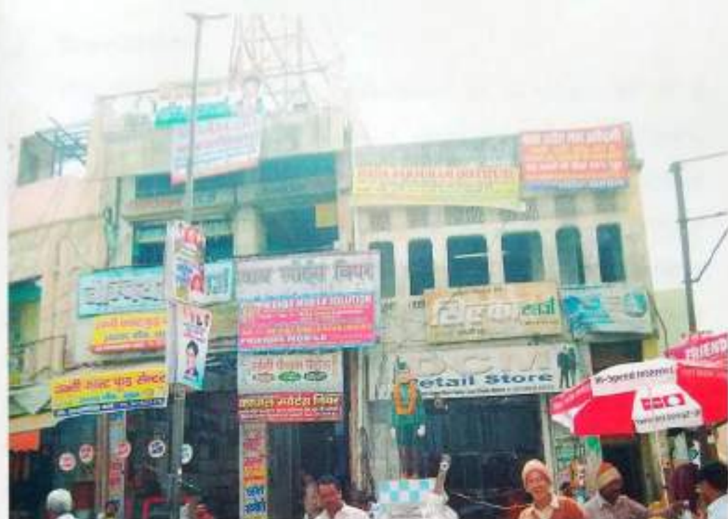
PLATE No 3.1 MULTI STORIES BUILDING IN MEHAM MARKET
